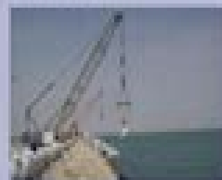
Placing Precast Sea Armour
