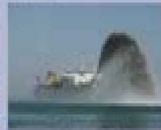
Reclamation by Spraying Sand
