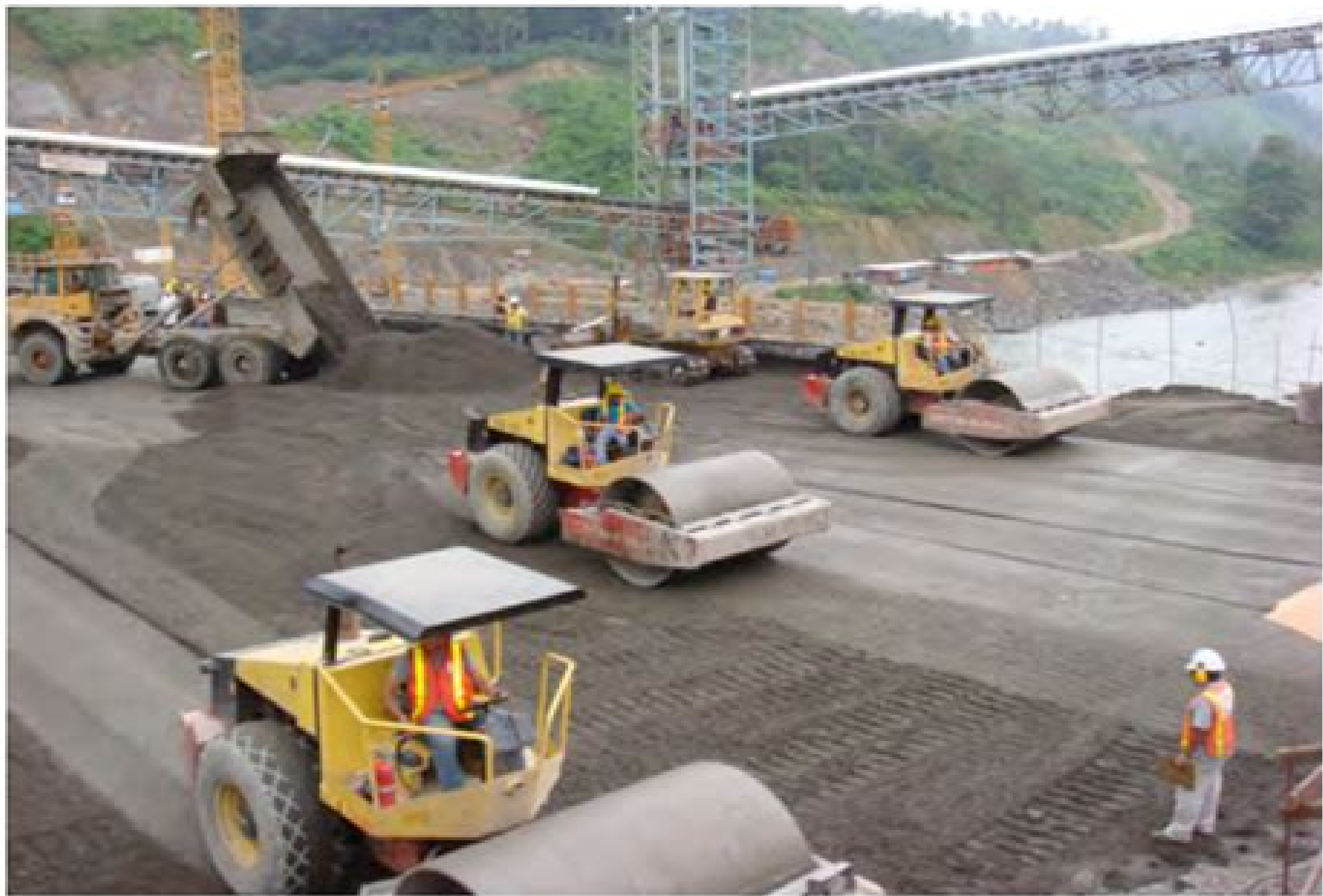
Figure 1. RCC dam construction
