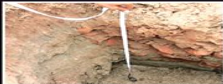
The Pavement composition is measured.
