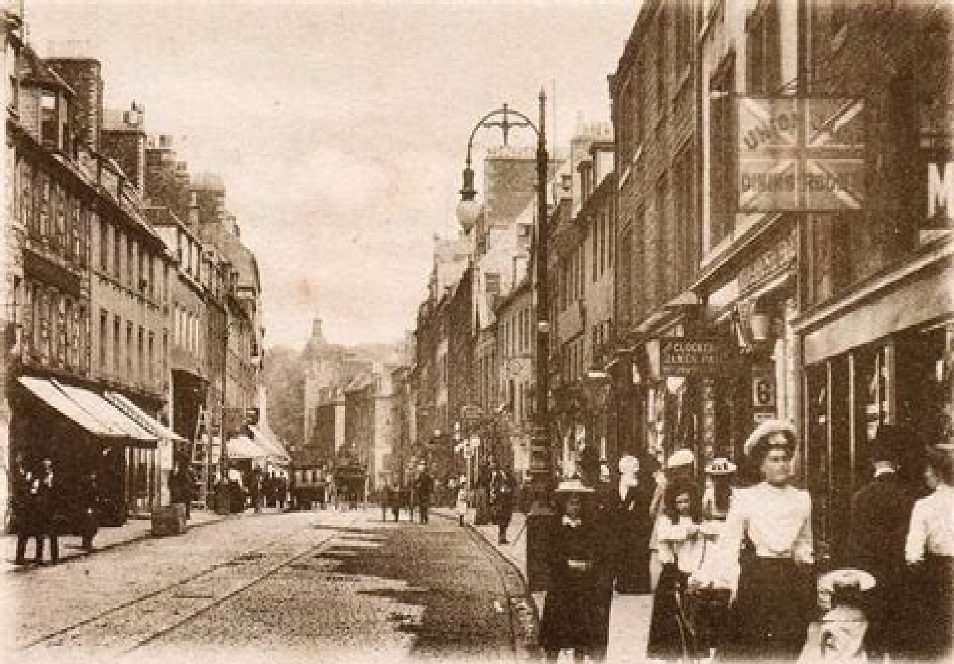
High Street, Perth, looking East.
