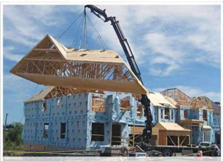
Each roof is lifted in sections and checked for square then is ready to be shingled.
