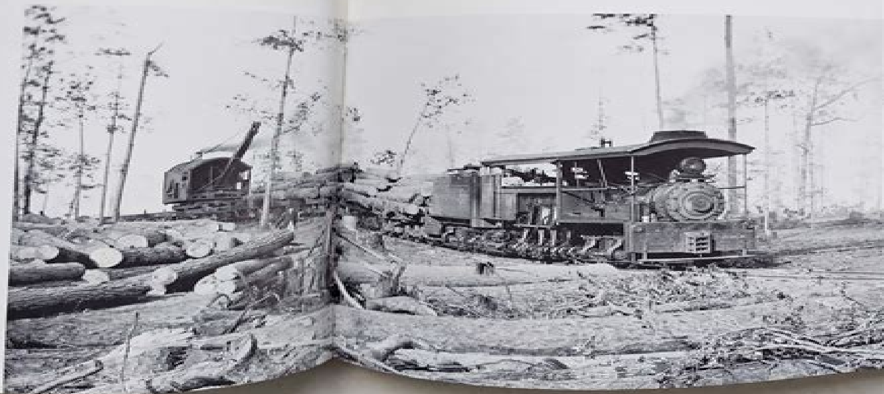
The operation of the Shay geared locomotive was limited to dry regions, in fact many locomotives exported for use around the world. On the left Shays of the J. I. Newman Lumber Co. shown at of hardwood at Newman's, Sumner, Mississippi station. At the lower left, the Philippine Insular Lumber Co. operated several Shay locomotives on their own line. Note the balloon stack and the large painted on the boiler smoke box for easy identification. There were many modifications applied to Shays, yet the most unusual might be the extended roof over the boiler of the Eastman, Gardner No. 62 at Laurel, Mississippi which is shown below.
