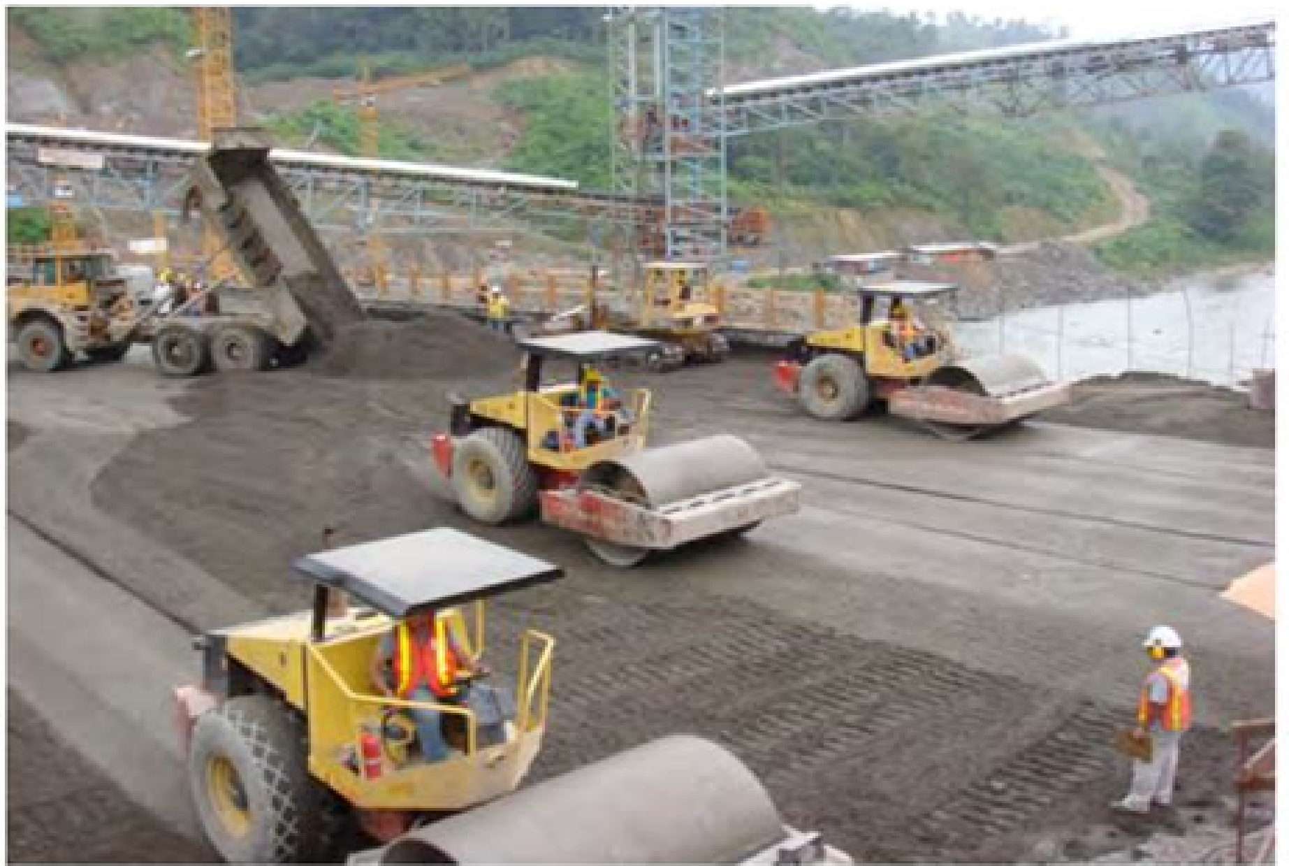
Figure 1. RCC dam construction
