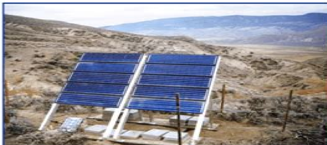
Figure 1 A Ten Panel Photovoltaic Array
