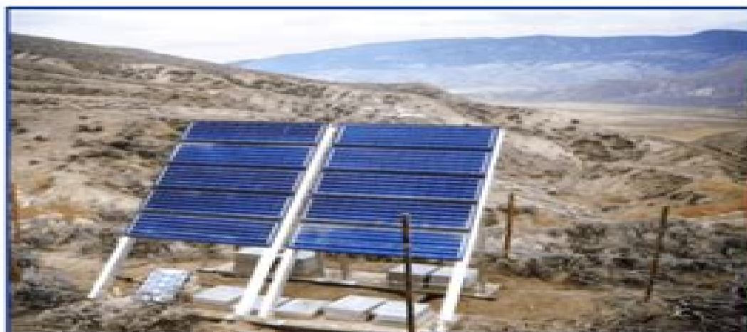
Figure 1 A Ten Panel Photovoltaic Array
