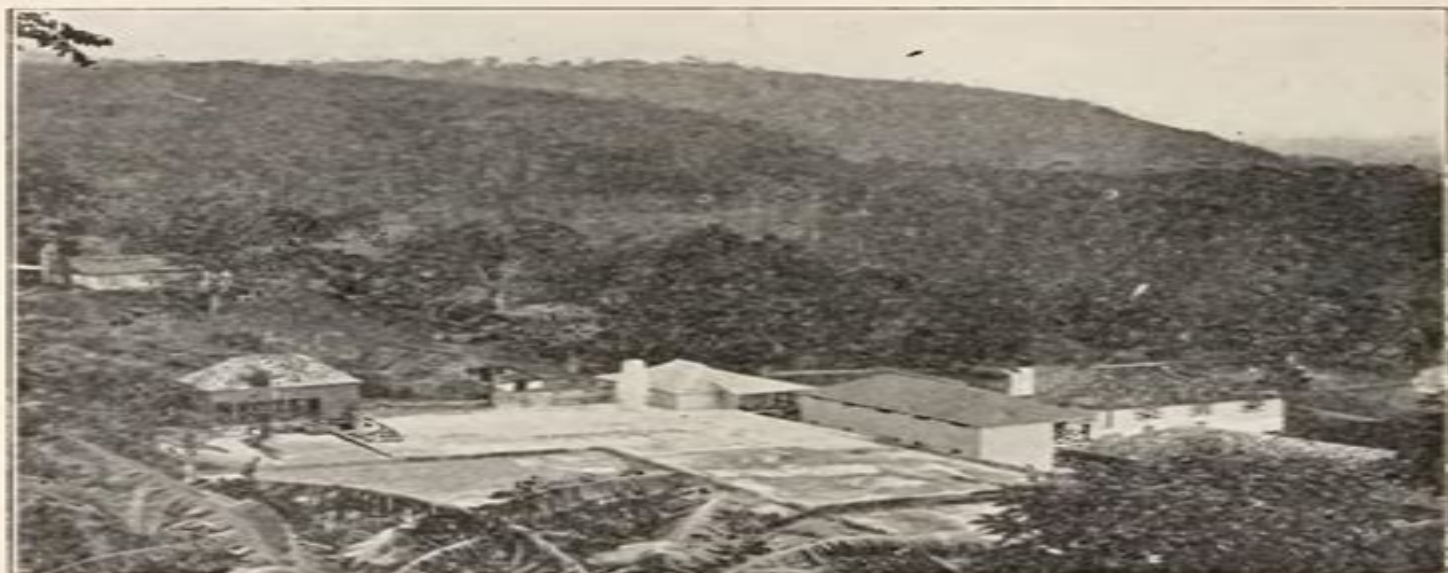
COFFEE PLANTER'S HOME WITH CEMENT DRYING FLOOR (BARBECUE). Pulping mill and windrows of drying coffee at left.
