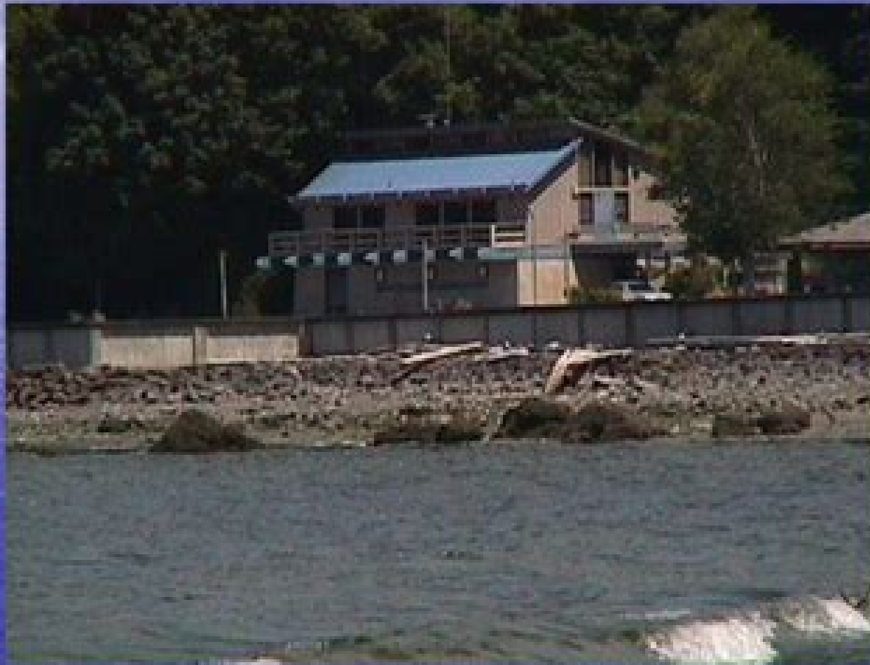
The Marine Technology Lab and Classroom at Seahurst Park
