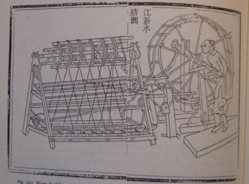
Fig. 247. Warp doubling and throwing-frame using the wet spinning method, Kiungsu-Chekiang (Chor. Che shai-fang thu), + 1899. TSTP, ch. 11, pp. 40ab.
