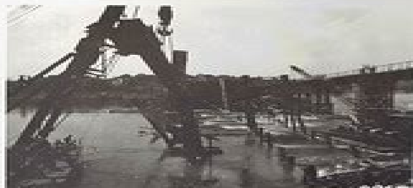
LIFTING STEEL; MAINZ
