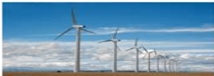
Above: Low weight and high strength makes FRP ideal for windmill blades.
